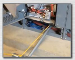
Using a standard 1" EMT pipe, the CP1000 can be extended to longer lengths for "hard to get to" areas such as under cabinets or panels and on ceilings or cross beams.
